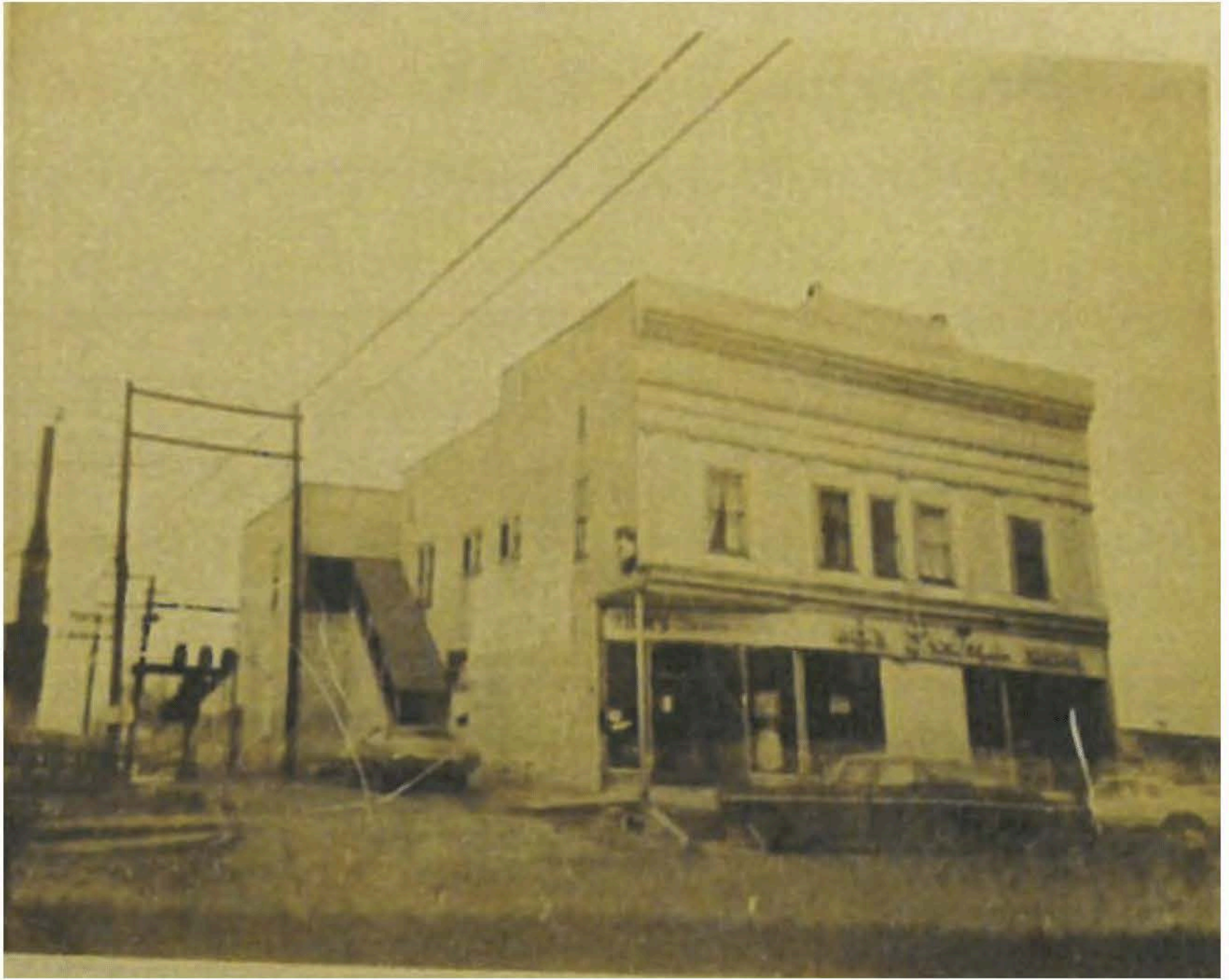
Figure 2-2: Circa 1960's photograph after alterations
