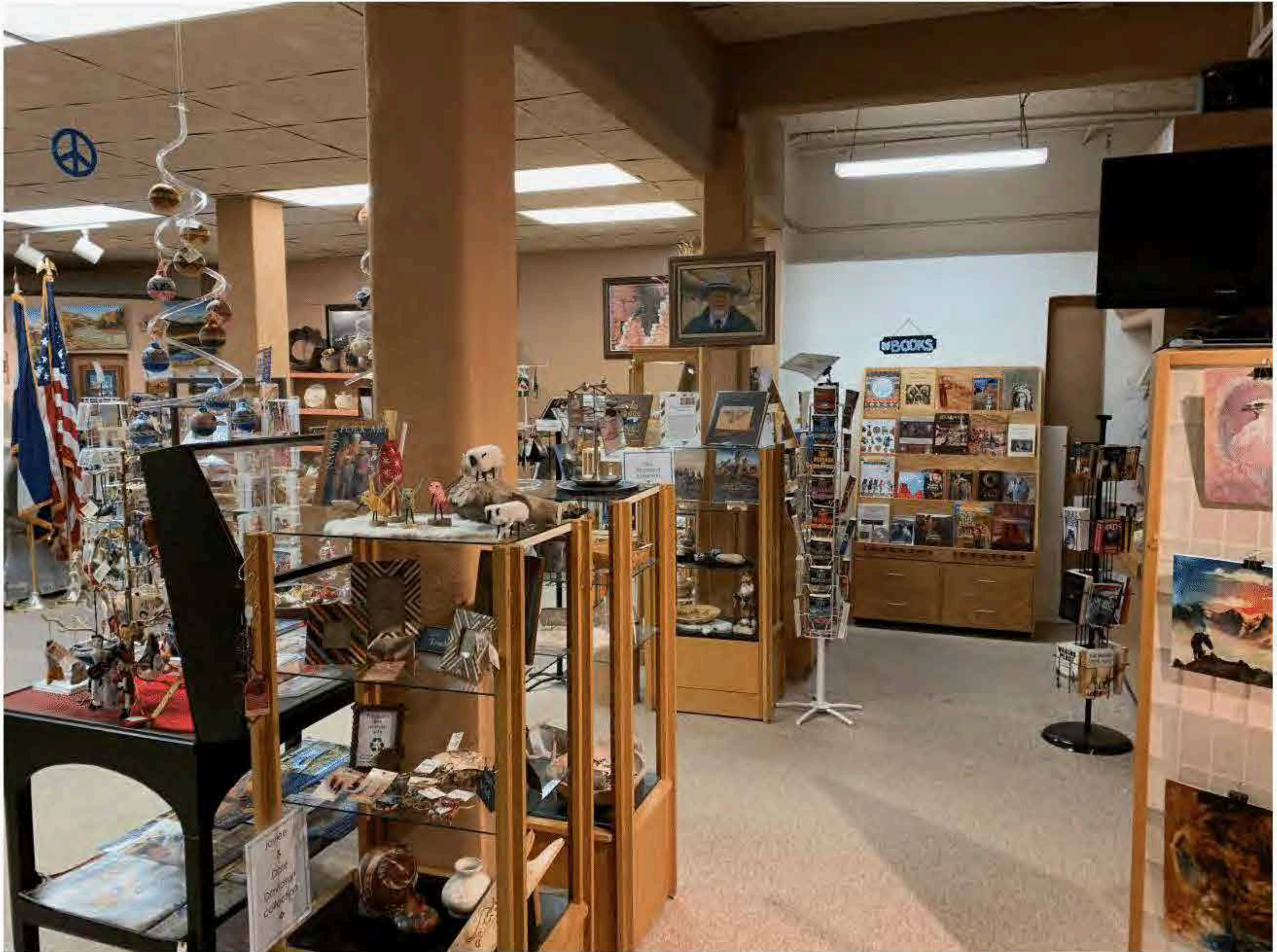
Figure 3.8-6: Main level dropped and grid mount fluorescent lighting
