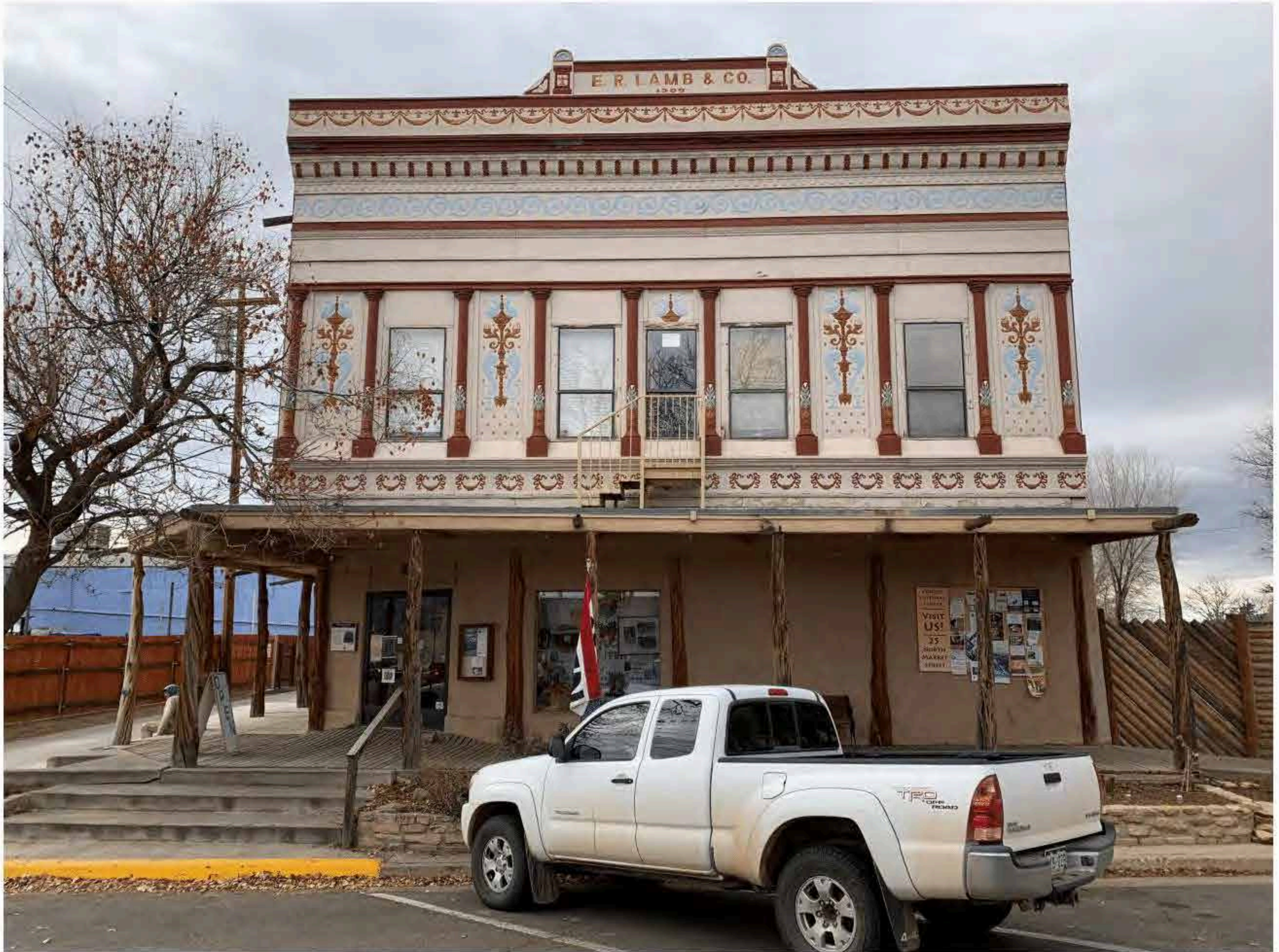
Figure 3.5-4: Current front facade and windows
