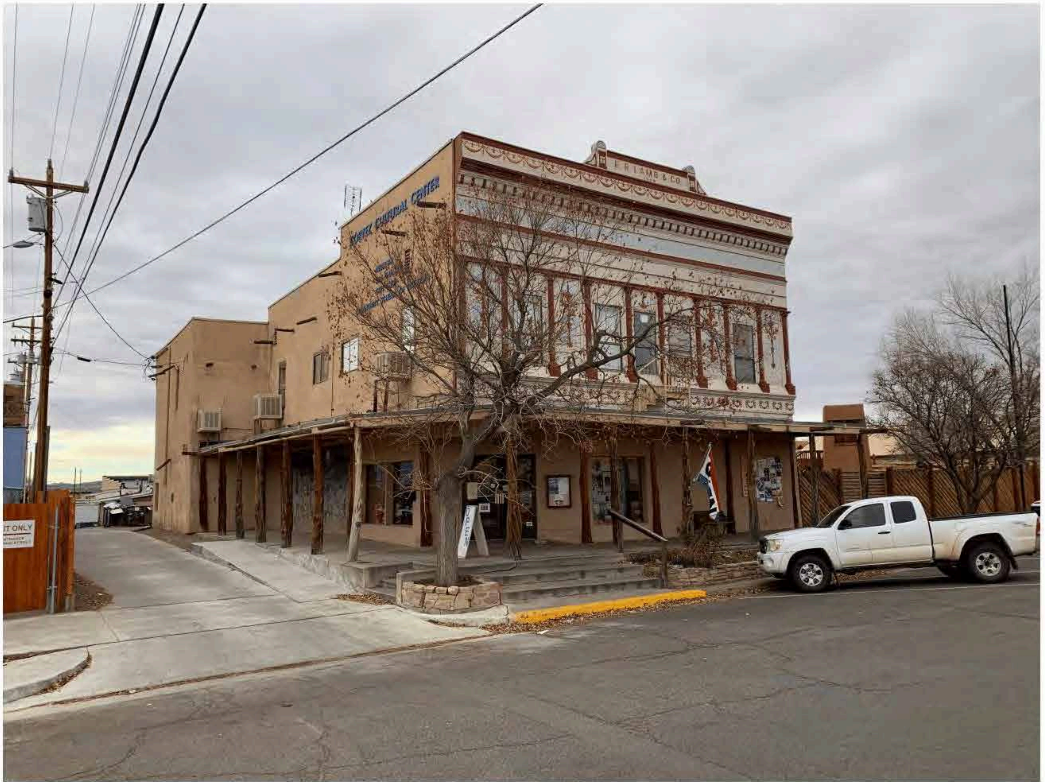
Figure 3.5-5: Current front and South facade and windows
