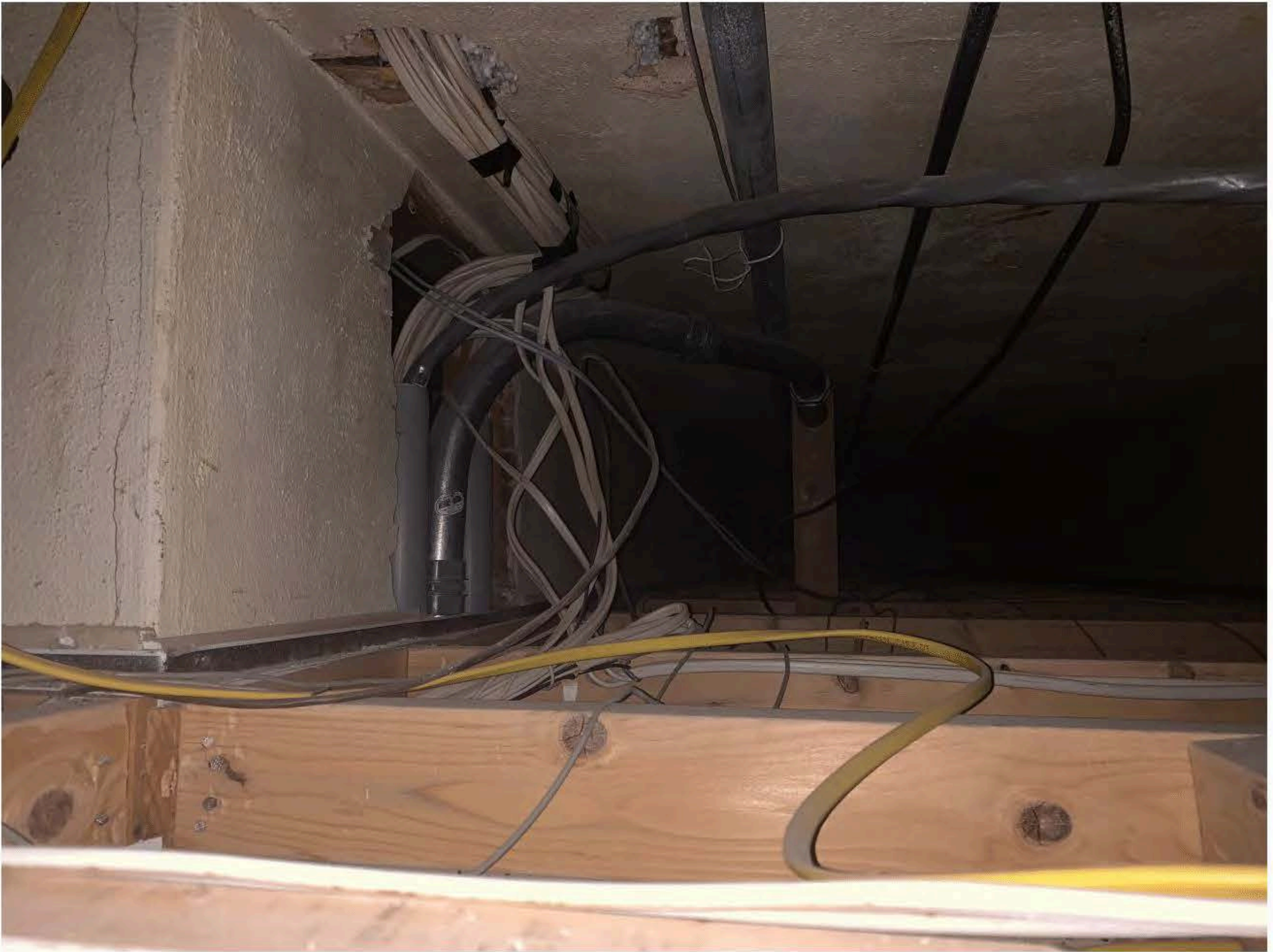
Figure 3.6-6: Dropped GWB ceiling and original lathe and plaster wall and ceiling
