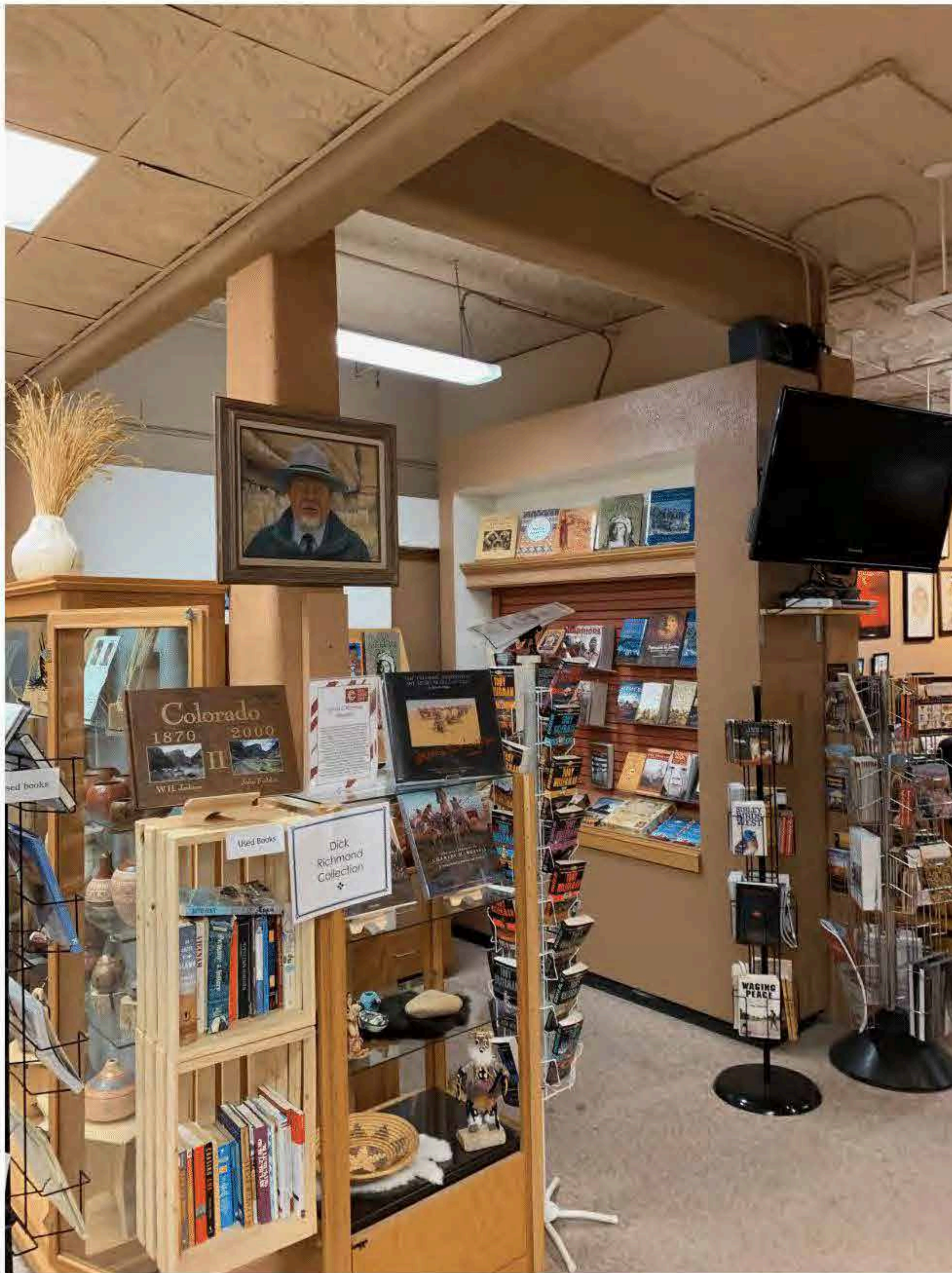
Figure 3.6-3: Typical stuccoed over beams, columns, and dropped ceiling
