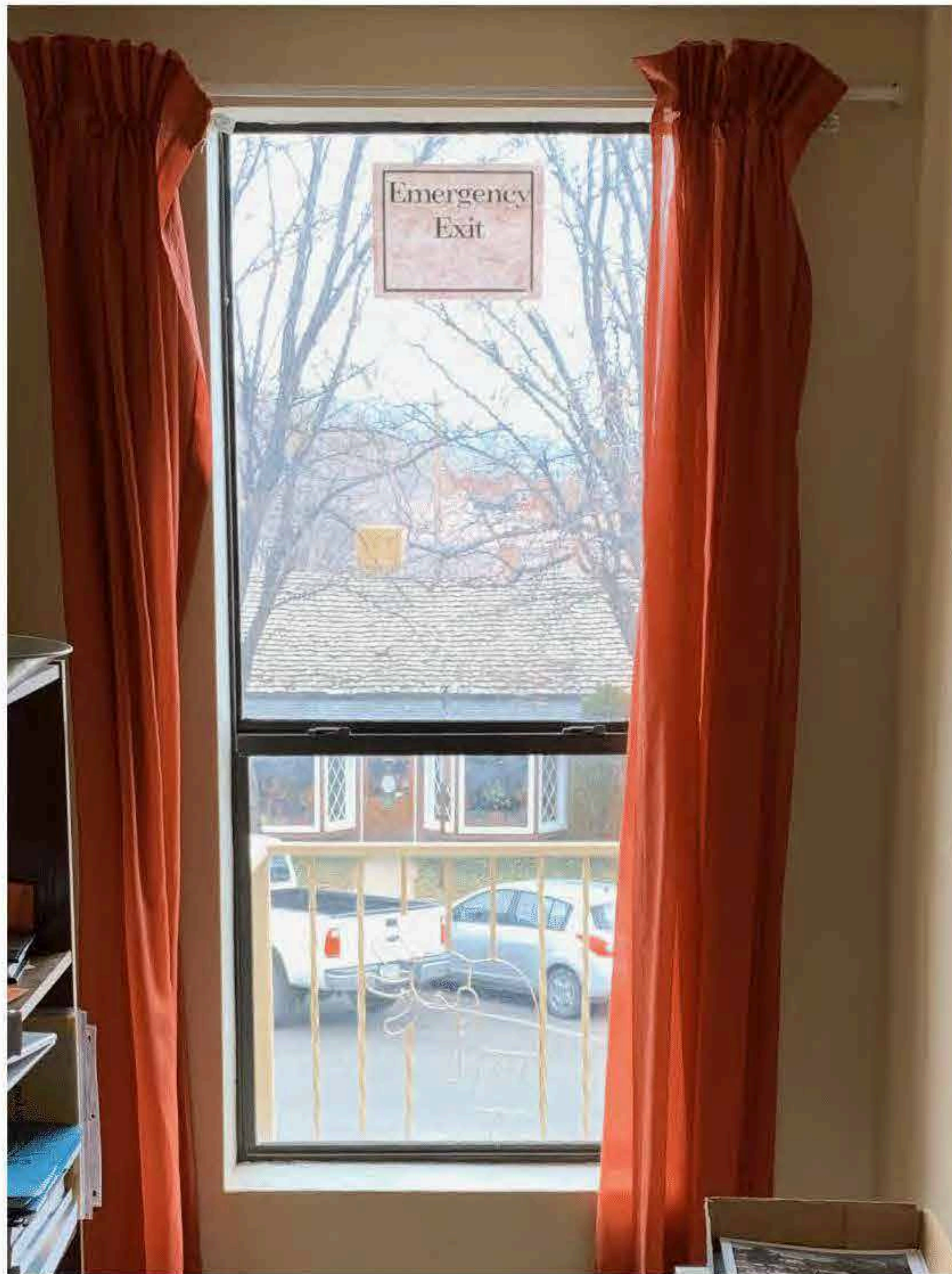
Figure 3.5-7: Current typical single hung aluminum window
