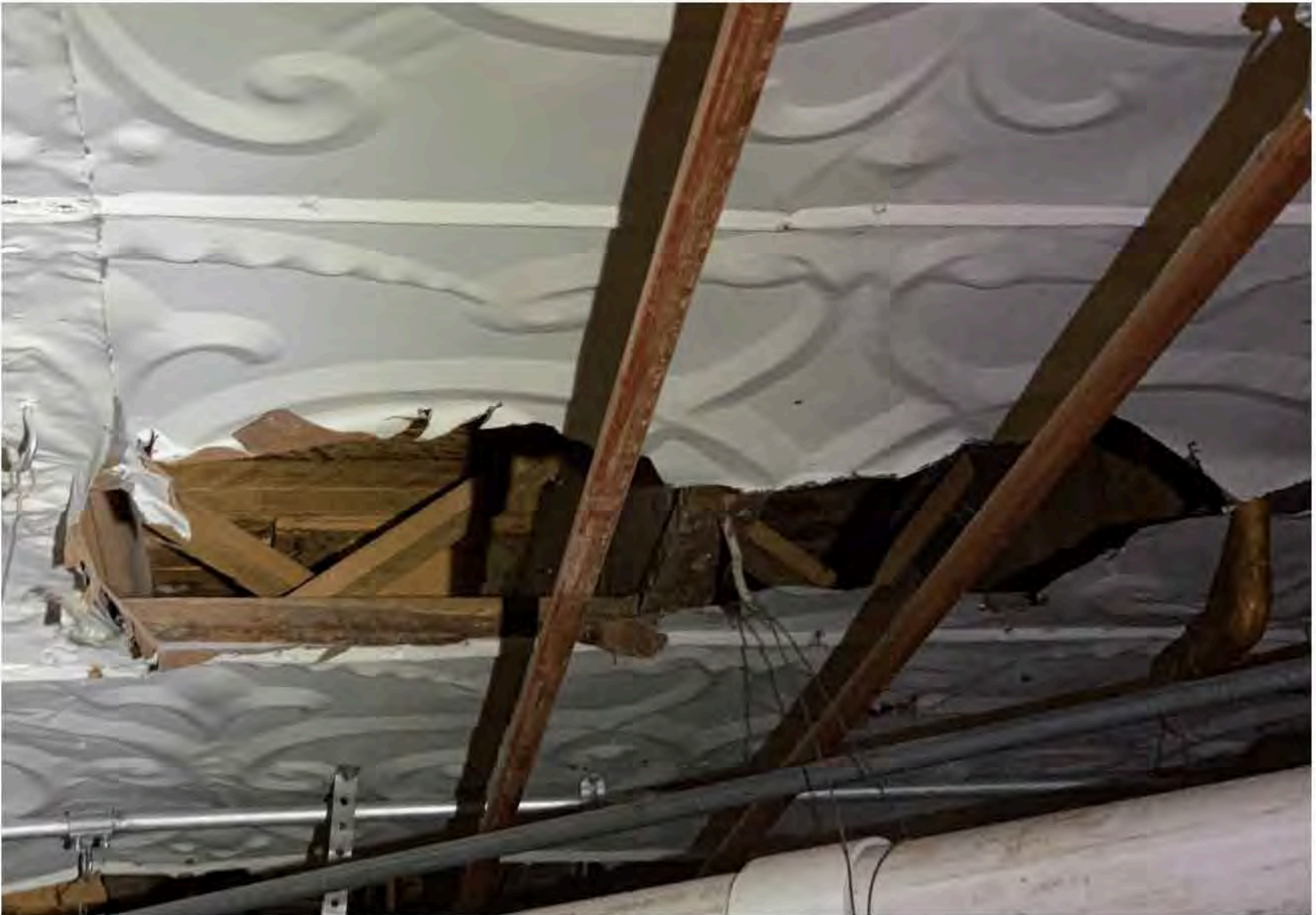
Figure 3.2-4: Glimpse of 2nd. level floor system
