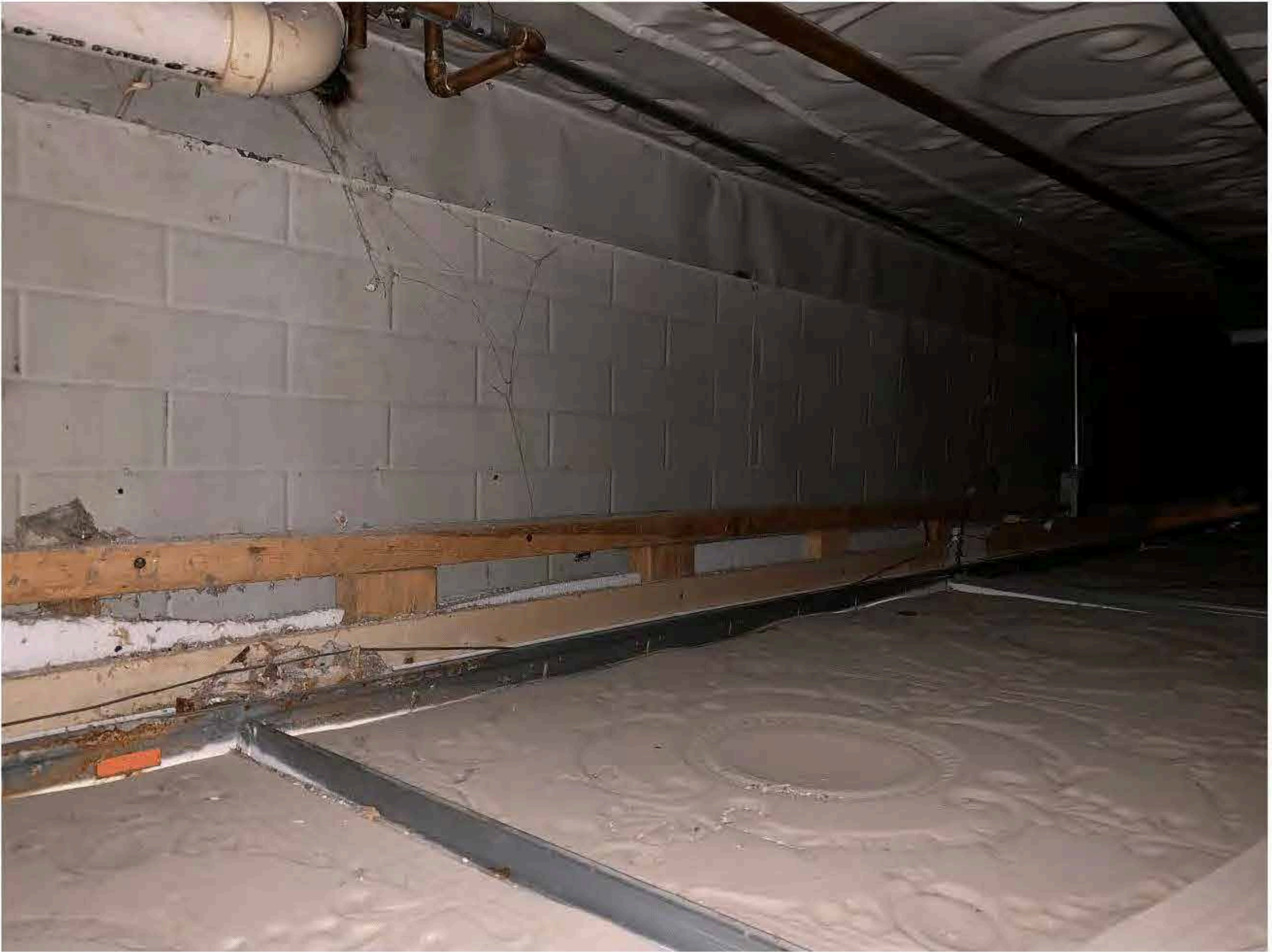
Figure 3.6-4: Dropped tin ceiling and original tin brick pattern wall
