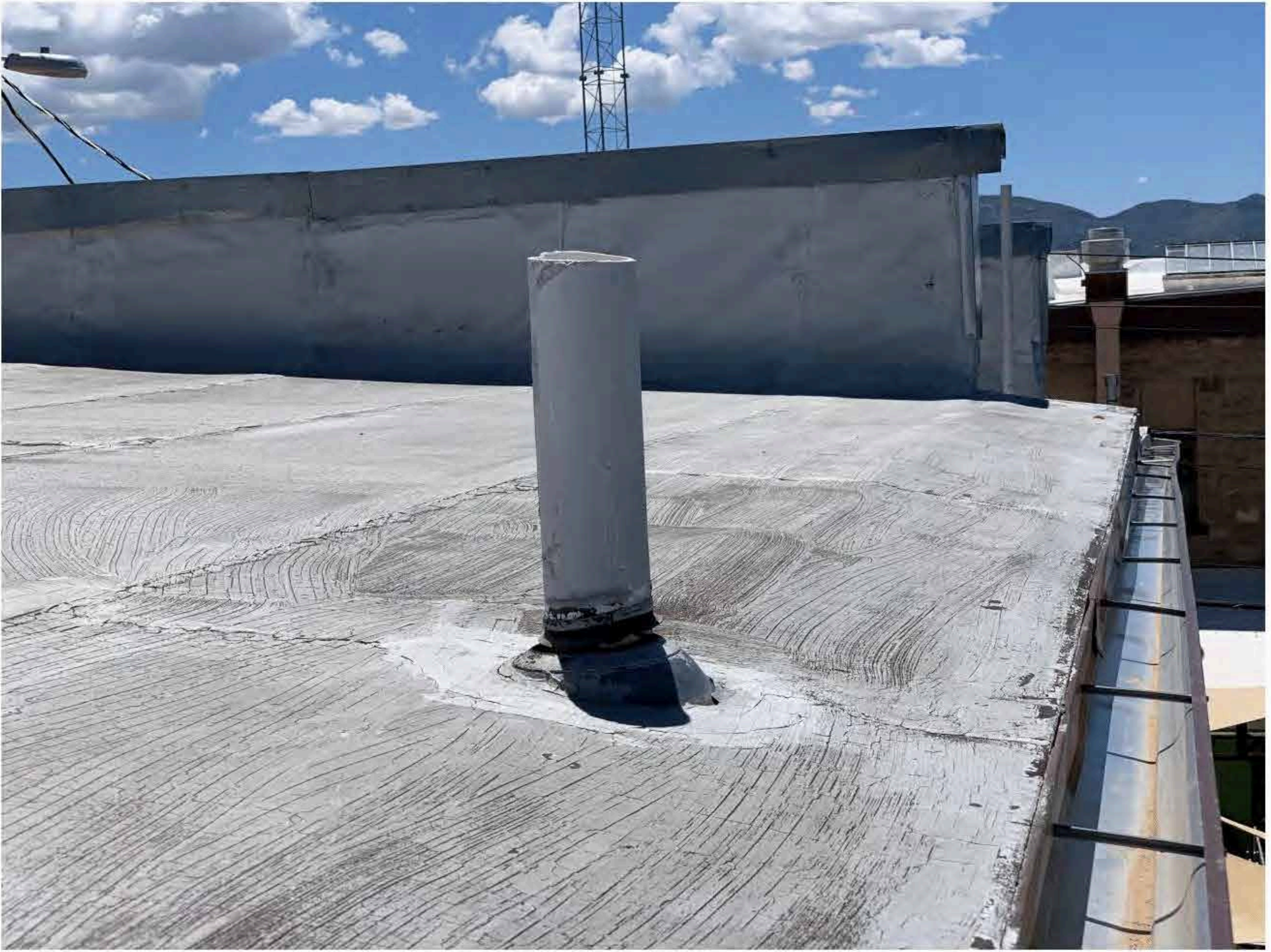
Figure 3.4-3: Main Roof at gutter looking South
