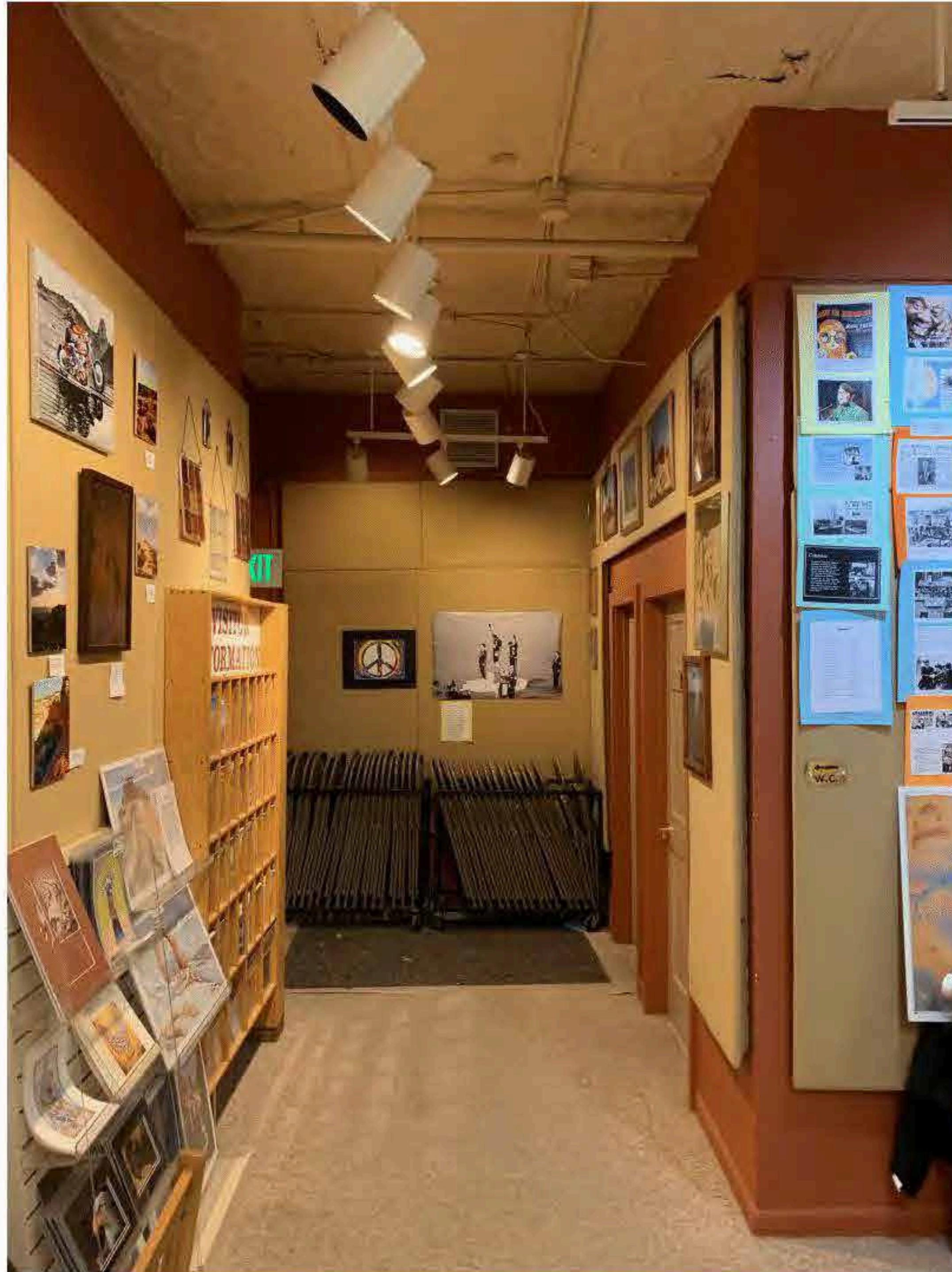
Figure 3.8-5: Main level surface mount track lighting
