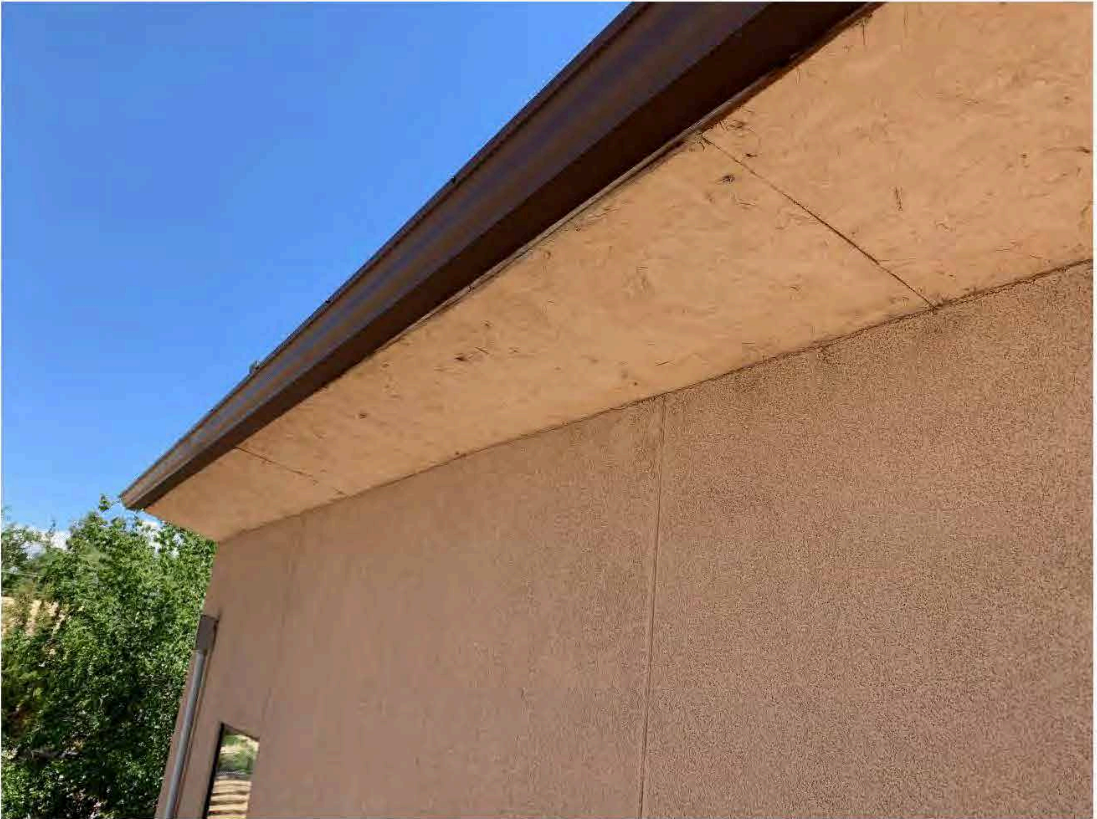
Figure 3.4-7: New OSB soffit
