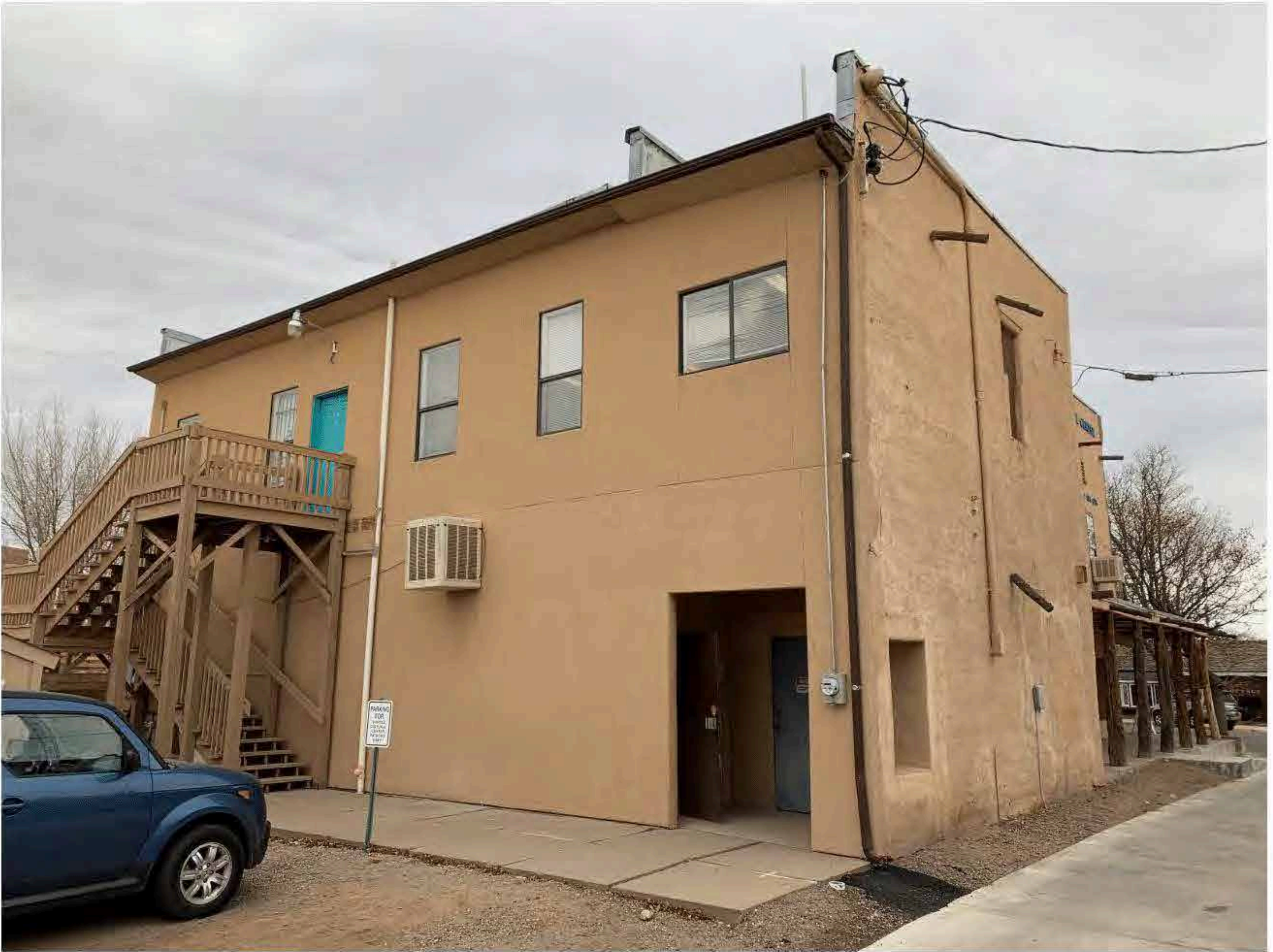
Figure 3.5-6: Current Southwest facade and windows
