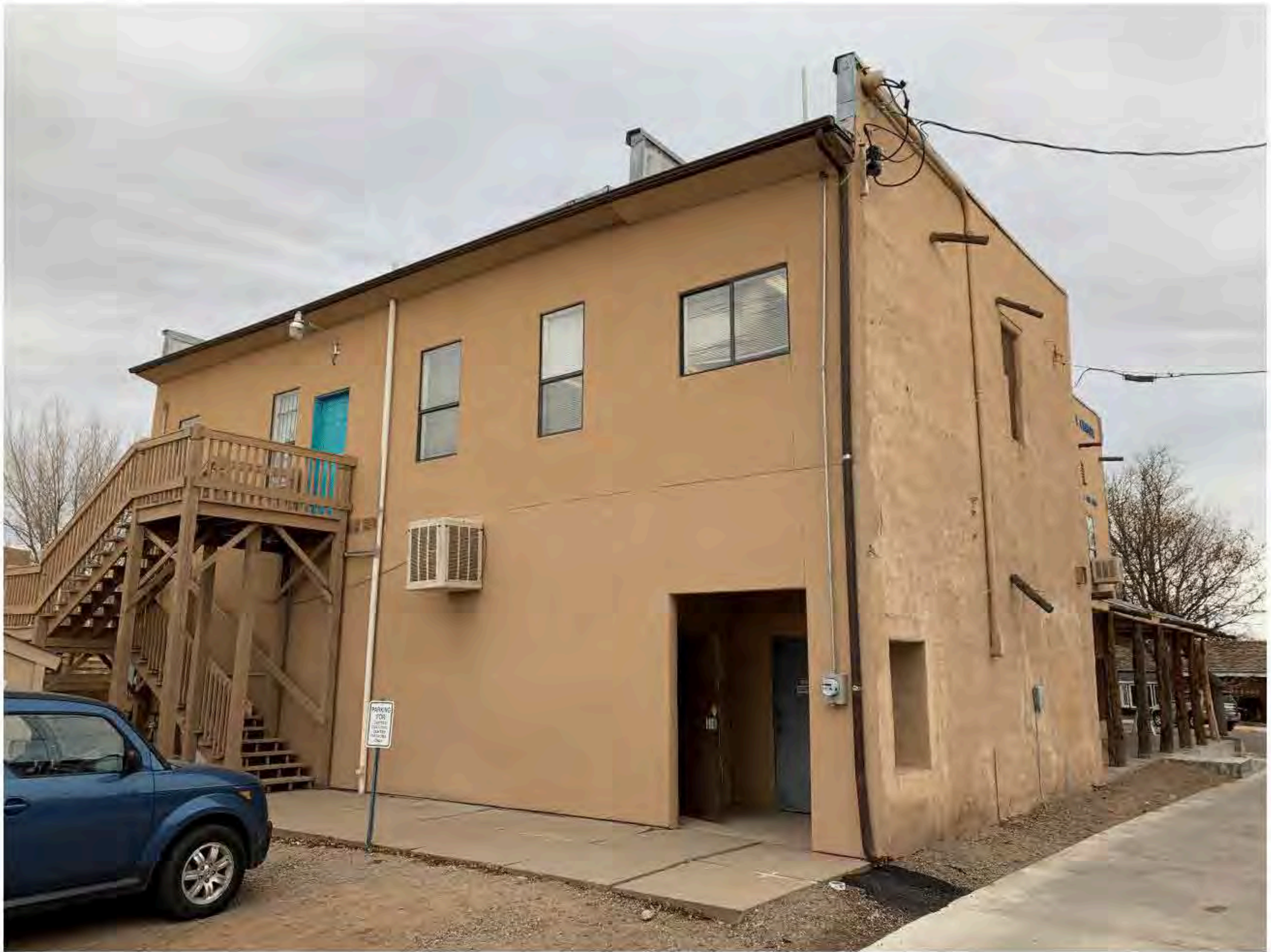
Figure 3.3-7: South and West facade
